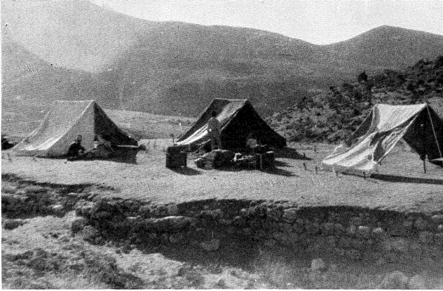
Fig. a. Camp at Shaikh'Adi on the roof of the old building. Seen towards SE
